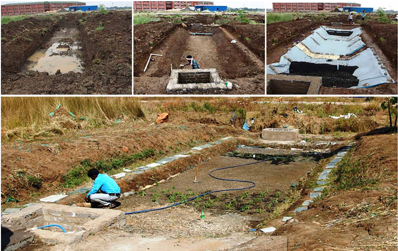
Figure 6 | Horizontal subsurface flow bed construction and implementation at IGNTU pilot plant.
